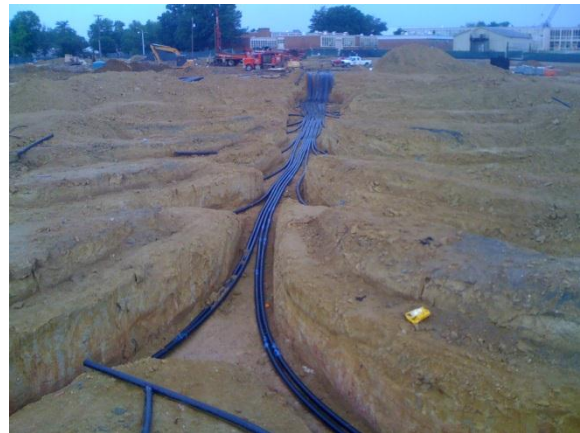
Figure 2: Horizontal Runs for Geothermal Wells
